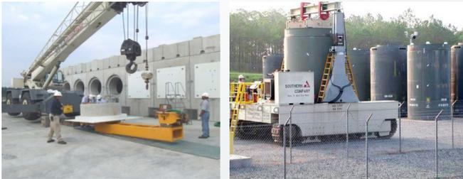
**Figure 1. A horizontal dry storage system, (left image) and vertical dry storage system (right image). Both of these systems use welded stainless steel canisters to contain the UNF.**
