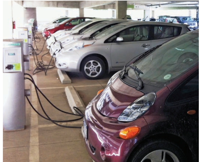
Electric vehicle charging stations at the STM campus parking garage. The 36 charging stations are part of a research project to test the impact of charging scenarios on the electrical distribution network. Use of electric cars has the potential to reduce carbon dioxide emissions that contribute to climate change. Photo by Erik Nelsen, NREL 26488
