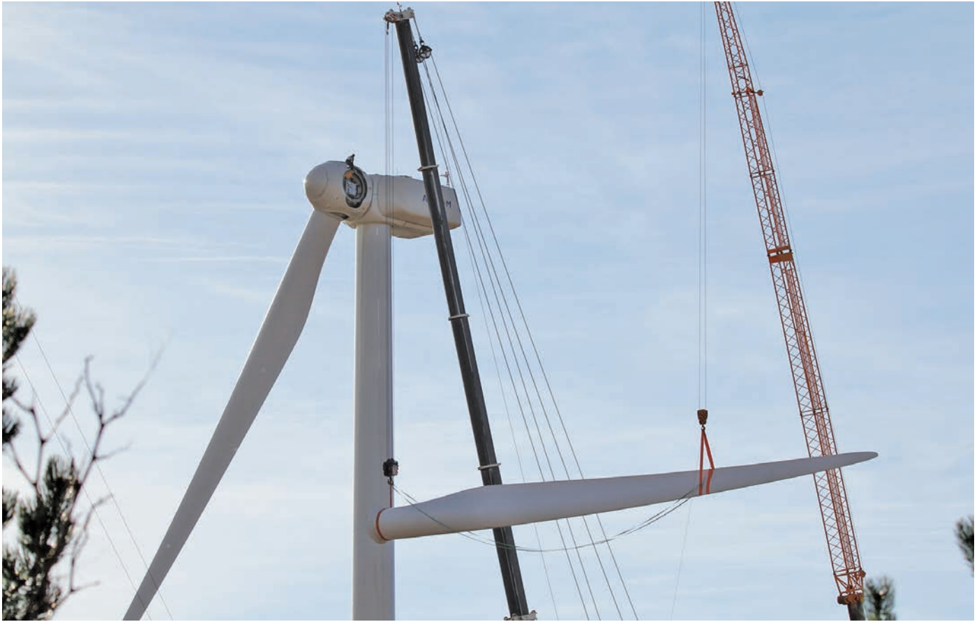
New blades are being installed for testing on a 3MW wind turbine at NREL's National Wind Technology Center. Photo by Lee Jay Fingersh, NREL 33210
