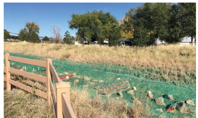
Improvements and erosion control measures at the Jeffco Swale. Photo by Karri Bottom, NREL 32736
