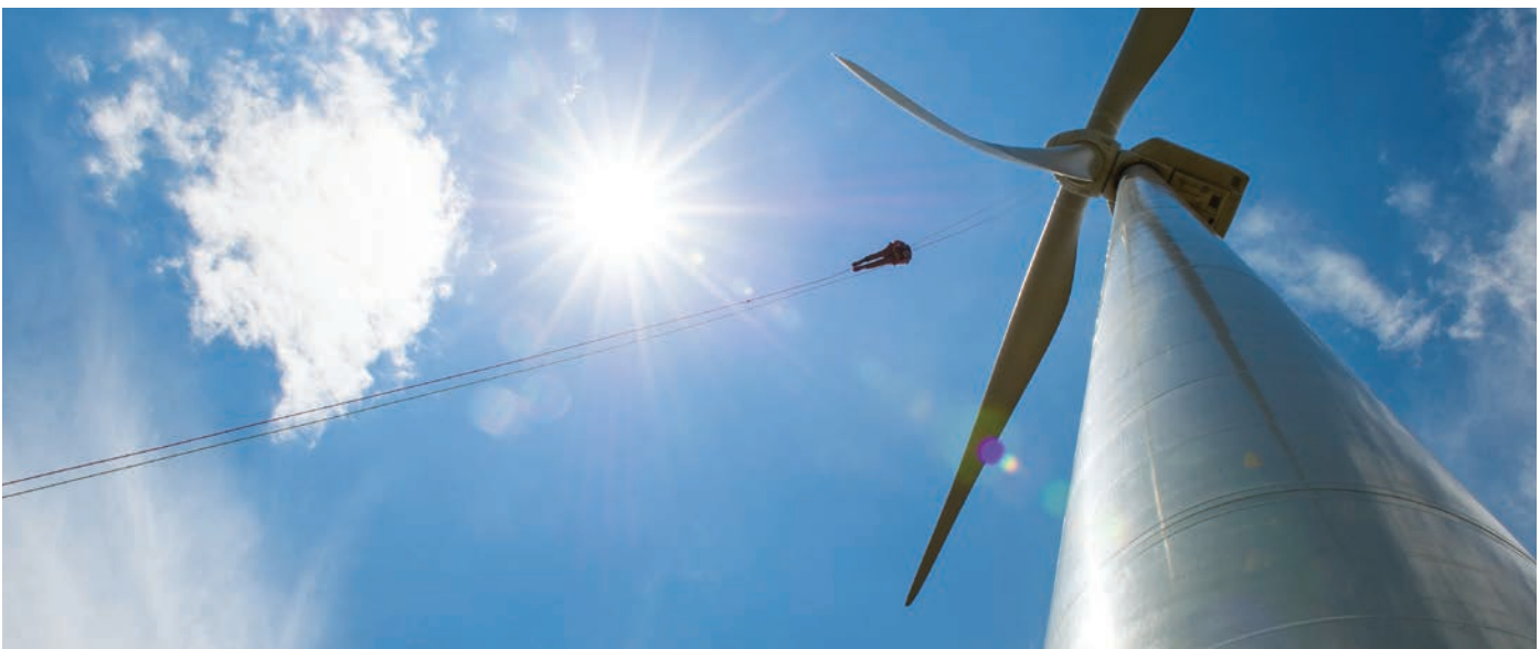
An NREL employee completes a blade inspection of a 3MW wind turbine at the NWTC campus. Photo by Dennis Schroeder, NREL 27198
