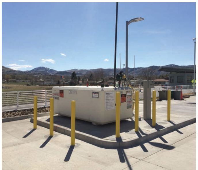
E85 fuel tank and fueling station at the STM campus. Photo by Larry Durbin, NREL 32761
