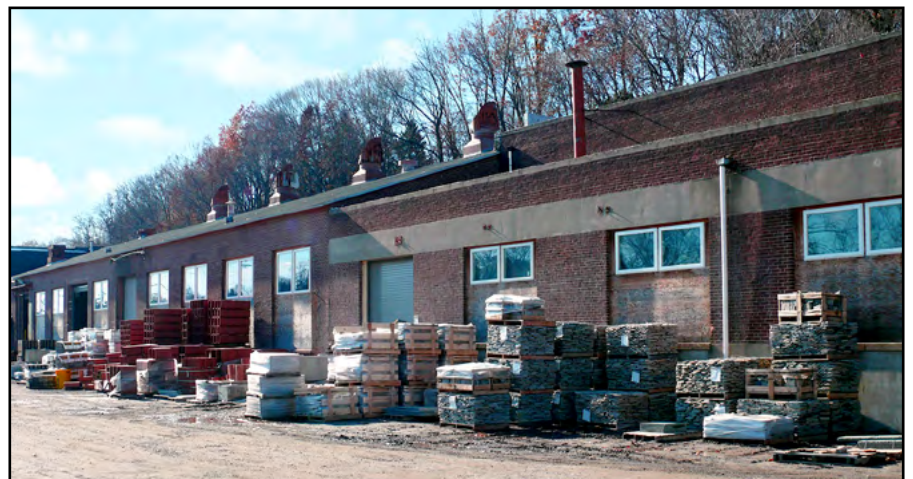
The Rufert building at the Seymour, Connecticut, Site is used to produce stone construction products, fire pits, and fireplaces (2014).
