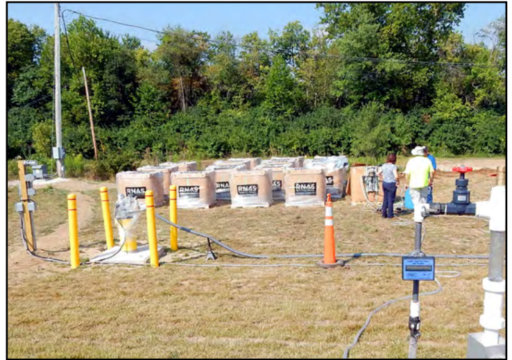
Totes containing emulsified oil are staged and ready for injection during the OU-1 field demonstration.
