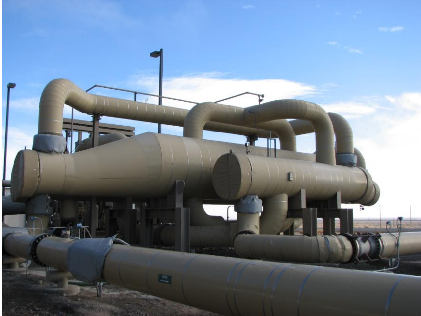
Dixie Valley Binary Plant
