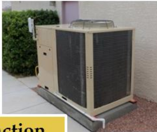
Multi-Function Gas-Fired Heat Pump
