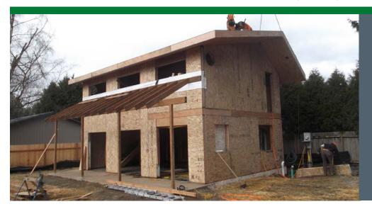
The walls and roof of the home were made of structural insulated panels consisting of two panels of OSB sandwiching a layer of rigid foam. The panels are precision cut in the factory and come to the site ready for quick assembly into a very sturdy, straight structure. The 6-inch-thick walls have an insulation value of R-26 while the 10-inch-thick roof has an insulation value of R-42.
