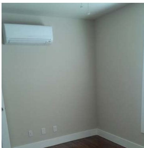
A high-performance ductless heat pump provides all of the home's heating and cooling.
