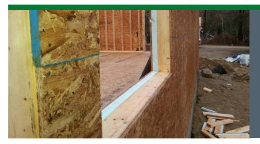
The home's walls are constructed with a 2x6 insulated stud product consisting of 2x4 lumber with 1.5 inches of extruded polystyrene (XPS) rigid foam glued to one end and covered with .5-inch OSB, which serves as a nailing surface on the inside of the wall. The rigid foam serves as a thermal break preventing heat transfer through the studs.
