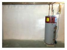
The home's heat pump water heater is located in the basement directly below the hot water fixtures on the first and second floors. The wall behind the water heater is covered with closed-cell spray foam painted with an intumescent ignition-barrier paint. The spray foam has a smooth hard surface similar to stucco.
