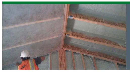
The cathedral roofs consist of engineered roof rafter I-joists that create a 14-inch space which is first air sealed with 1 inch of closed-cell spray foam then filled with blown cellulose for a total attic insulation value of R-60.
