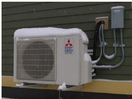
A single one-ton mini-split ductless heat pump (outdoor unit shown here) was enough to heat and cool the entire 1,650 ft<sup>2</sup> two-story home. A small duct with an inline fan helped pull conditioned air through the ceiling to upstairs bedrooms. An ERV provided fresh air ventilation and also helped to circulate conditioned air with a supply duct in the great room and return ducts in the bedrooms and bathrooms.
