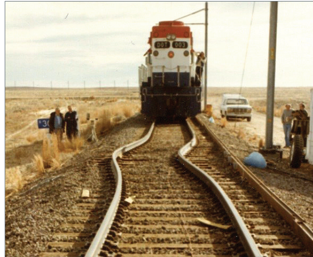
Figure 2-9. Rail Thermal Misalignment 135
