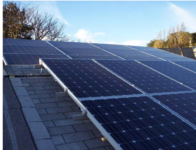
19 PV Panels, 320 Watts Each, South Facing
