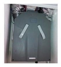
An innovative HVAC solution using a single mini-split indoor unit and a heat recovery ventilator (HRV) supplies air directly to a great room. A separate compact distribution system with a single efficient fan exhausts air from the great room and delivers it to the bedrooms. This cost-effective strategy can provide space conditioning in small-to medium-size low-load homes.
