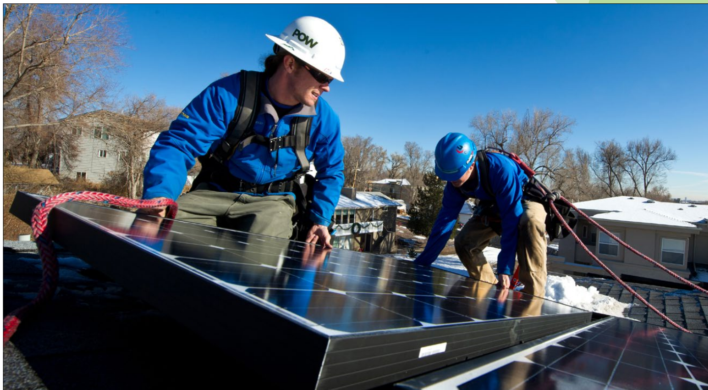
Solar energy's growth is demonstrated here as Kyle Travis (left) and Jon Jackson (right) with Lighthouse Solar install microcrystalline PV modules on top of a town home. By 2014, solar PV installations were about 15 times what they were in 2008 (SEIA and GTM Research, 2014). Photo by Dennis Schroeder, NREL.
