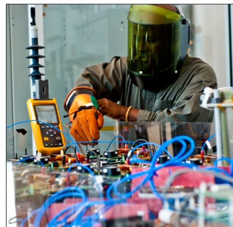
Smart grid work in progress at the FREEDM Systems Center at North Carolina State University (NCSU). Photo courtesy of NCSU.
