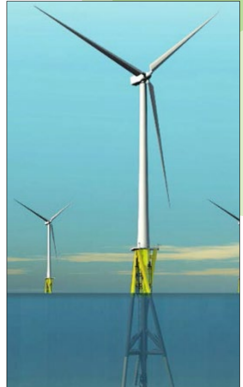
Both Dominion Virginia Power and Fishermen's Energy will use a twisted jacket foundation, where three legs are twisted around a central column. Photo courtesy of Fishermen's Energy.
