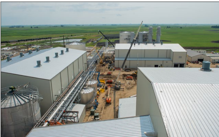
The mechanical building (front), solid/liquid separation (left) and anaerobic digestion areas (back) at POET-DSM’s Project LIBERTY biorefinery in Emmetsburg, Iowa. Photo courtesy of POET-DSM.
