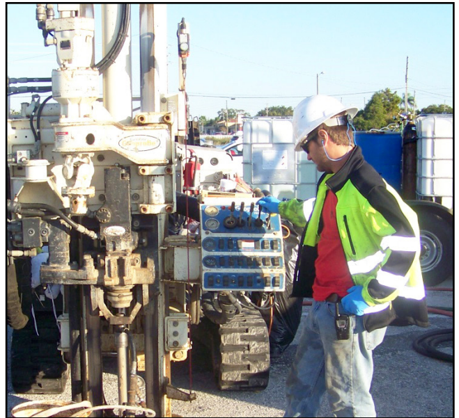
A contractor uses a direct-push rig to inject emulsified vegetable oil (EVO) and Dehalococcoides mccartyi into the soil. The transfer tanks containing the EVO are in the background.
