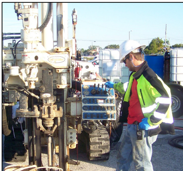
A contractor uses a direct-push rig to inject emulsified vegetable oil (EVO) and Dehalococcoides mccartyi into the soil. The transfer tanks containing the EVO are in the background.
