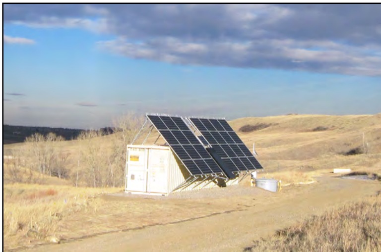
Figure 2. Air stripping at the East Trenches Plume Treatment System focused on water that was not yet treated using iron filings. The spray nozzles (above left) are located in the gray manhole next to the solar array shown in the photo on the right. The solar panels charge batteries located inside the conex, which power the pump.
