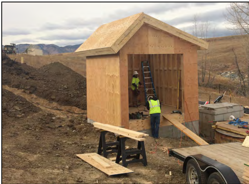
Figure 3. The new, commercial air stripper is shown in the left photo above, and will be housed in the shed shown in the photo on the right. The roof of the shed is angled to provide better solar-thermal exposure. The solar/battery conex from Figure 2 (see page 14) is visible in the background to the left of the shed.
