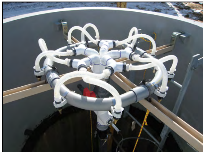
Figure 2. Air stripping at the East Trenches Plume Treatment System focused on water that was not yet treated using iron filings. The spray nozzles (above left) are located in the gray manhole next to the solar array shown in the photo on the right. The solar panels charge batteries located inside the conex, which power the pump.
