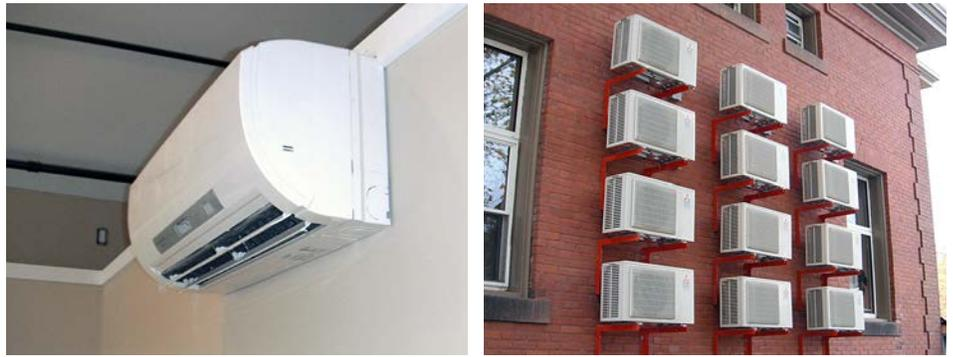
Ductless heat pumps provide most of the heating and cooling for the apartments. Finding room for all the outdoor units was a challenge; most were tucked on the rear wall of the building.
