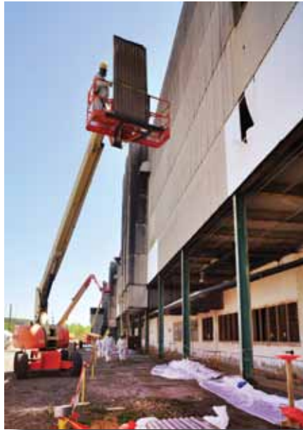
Workers remove paneling from the K-31 Building at ETTP in preparation for demolition in FY 2015.
