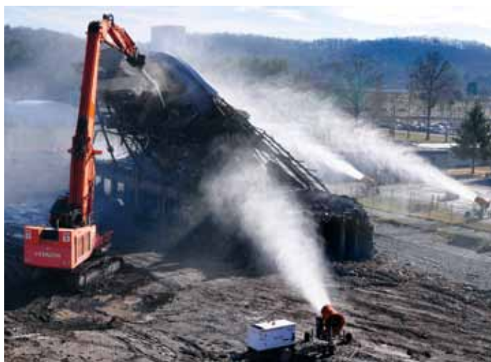
DOE reached a major milestone in December 2013 with the demolition of the last section of the K-25 Building at ETTP.
