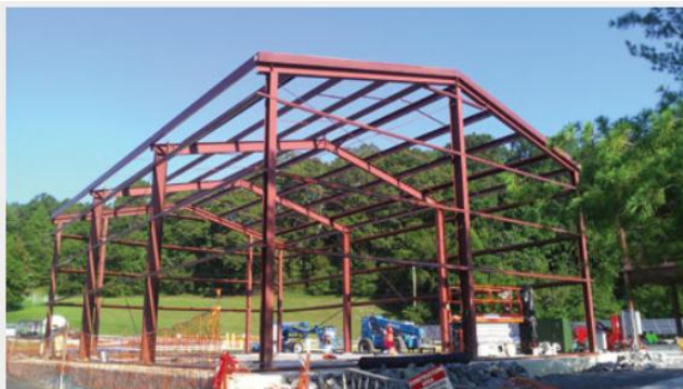
The skeletal framing for the low-rise FRP building.
