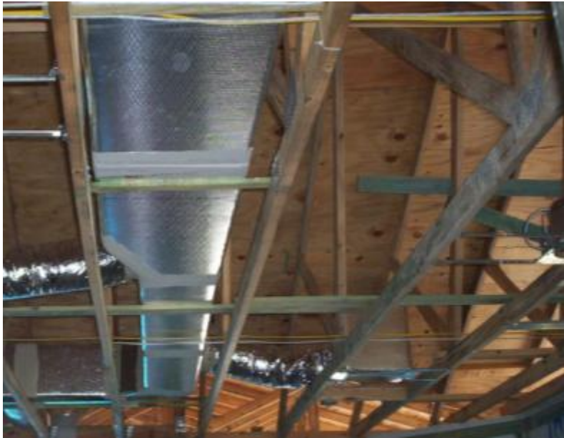
■ Before ceiling drywall
