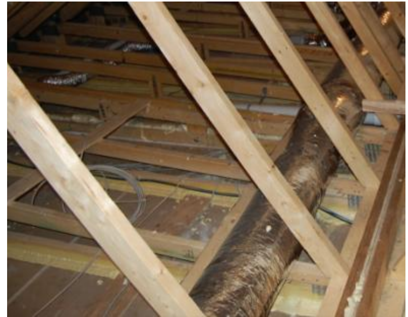
■ After ceiling drywall
