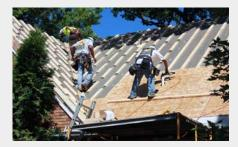
Short (2-in  $\times$  4-in.) sleepers are placed over the insulation to create cross ventilation in valleys before the roof decking is added.
