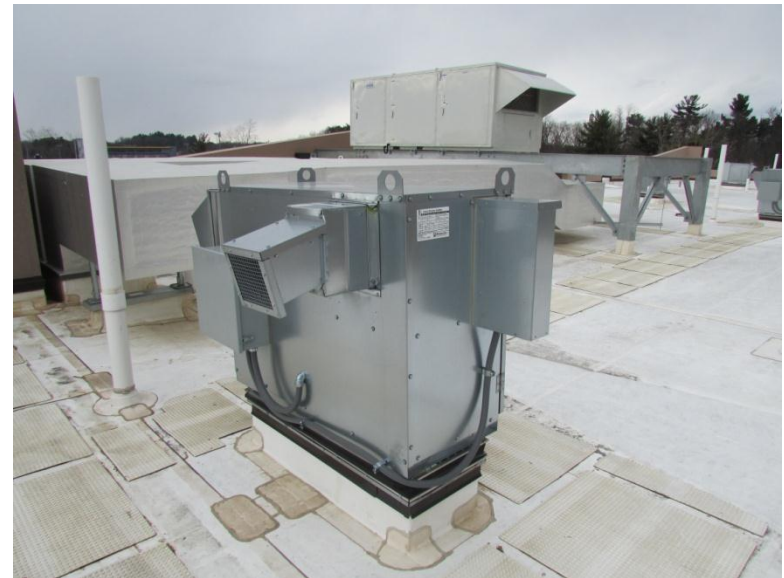
Improperly Conditioned OA Ventilation
