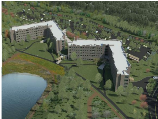
Student Housing at University at Albany with a Distributed GSHP system
