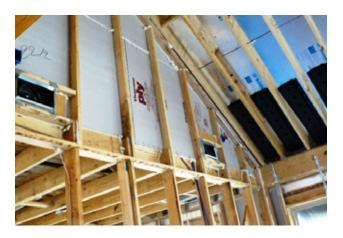
Advanced framing, which includes aligning all framing elements from the roof to sill plate, saves lumber. The savings more than offset the cost of additional insulation. The roof sheathing is lined with a radiant barrier to reduce solar heat gain for additional energy savings.
