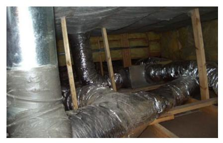
The builder worked with Building Science Corporation to design an insulated attic to provide a protected environment for the home's air source heat pump and ducts.
