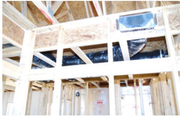
Artistic increased the efficiency of its heating and cooling systems by putting ducts in conditioned space in a central chase down the main hallway.
