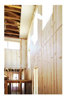
The 2x6, 24-inch on-center advanced-framed walls are stuffed with R-23 of blown-in fiberglass while an additional R-7.5 of rigid insulation wraps the exterior, providing a total wall insulation value of R-30.5.
