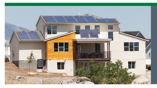
The DOE Zero Energy Ready Home is loaded with solar panels to take advantage of Utah's sunny weather. The 10.29-kW photovoltaic system more than meets the home's electric needs while the solar water heating panels are sized to meet the majority of the home's hot water needs.
