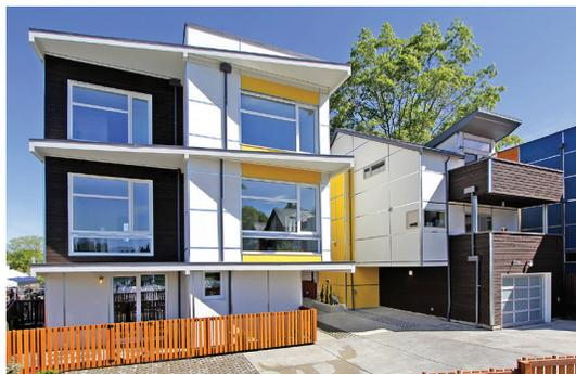
The flat roofs provide an ideal location for rooftop decks and solar panels, supported by 18-inch trusses that provide space for a combination of 2 inches of closed-cell spray foam and more than 16 inches of blown cellulose delivering a total insulation value of R-60. Double-stud 14-inch-thick walls allow for R-45 of blown cellulose.
