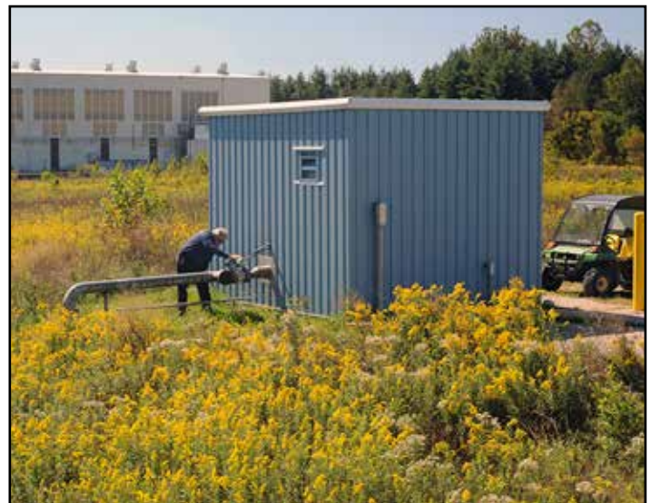
Groundwater remediation efforts at Fernald Preserve account for more than 80 percent of LM’s energy usage. Recently installed electric metering capabilities at each extraction-well house helped LM hit its metering goals. The system’s extraction wells and pumps receive routine maintenance by a small staff of contractor employees.
