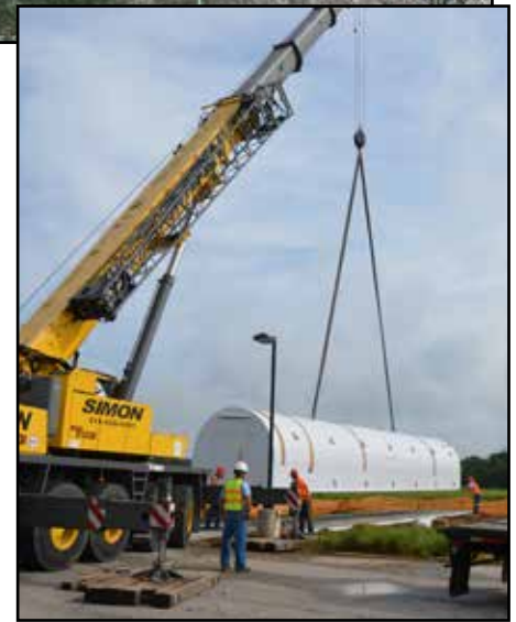
Shelter being placed on a concrete slab.
