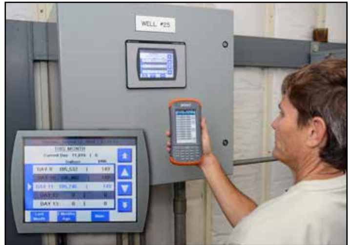
The new well-field control system at Fernald Preserve has reduced energy usage at the site, helping LM meet Executive and DOE energy use goals. Wireless functions within the system allow system monitoring for increasing efficiencies.
