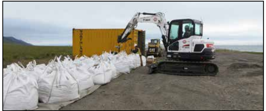
Super-sacks are weighed before being placed in Conex containers. The Conex containers were removed by barge to a permitted offsite disposal location.
