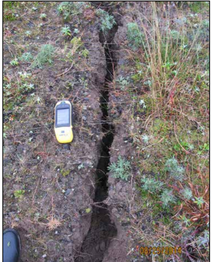
After 2014 earthquake—a crack along the northeast side of cap at the Long Shot Site is documented (August 2014).
