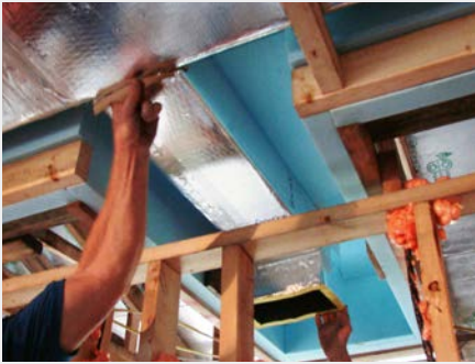
Lateral duct with chase running between trusses. Duct size is limited.
