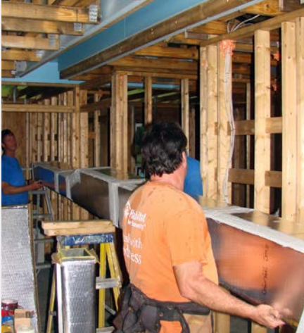
Main duct is lifted into place.
