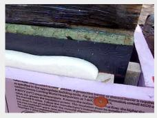
XPS foam is used in conjunction with the liquid foam above grade. It holds the foam in place and provides a smooth surface for a parge coat.
