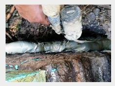
The liquid foam is easily applied in the trench. It conforms easily to the space below and strongly adheres to rough, uneven surfaces.
