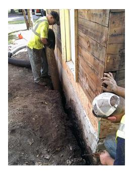
The excavationless process uses hydrovac technology to cut a precise 3–4 in. wide trench to a desired depth. The pressurized water loosens soil around the foundation while the vacuum extraction process removes the water-soil slurry. Once clean, the trench can be filled with liquid foam insulation.
