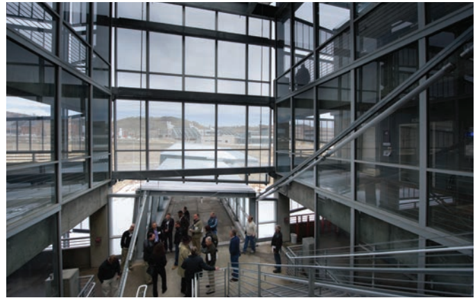
The glass at the parking garage is bird-friendly with vertical frits to prevent collisions. Photo by Dennis Schroeder, NREL 24898
