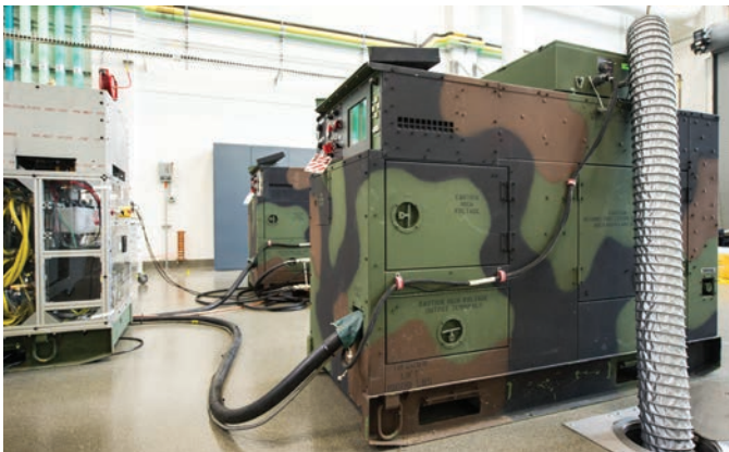
Consolidated Utility Base Energy System is an integrated power electronic platform for a 60-kW PV-Battery-Diesel hybrid power system developed for the U.S. Army to provide power to Forward Operating Bases. Photo by Dennis Schroeder, NREL 28837
