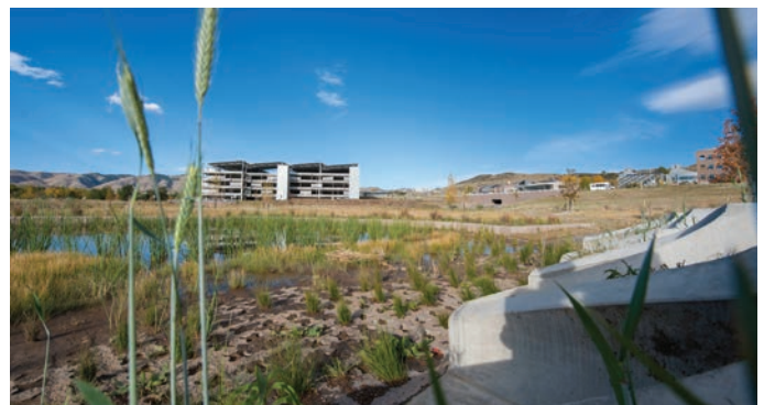
The STM stormwater detention pond regulates the flow of stormwater from the STM campus to neighboring Lena Gulch, mimicking pre-development hydrology. Photo by Dennis Schroeder, NREL 23189
