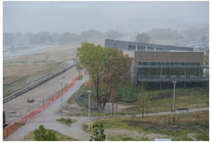
Resurfacing of Denver West Parkway with concrete pavers during the historic rainfall event of September 2013. Photo by Dennis Schroeder, NREL 27635
