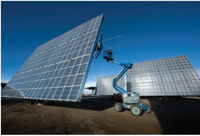
CPV array at SolarTAC in Aurora, Colorado. Photo by Dennis Schroeder, NREL 25538
