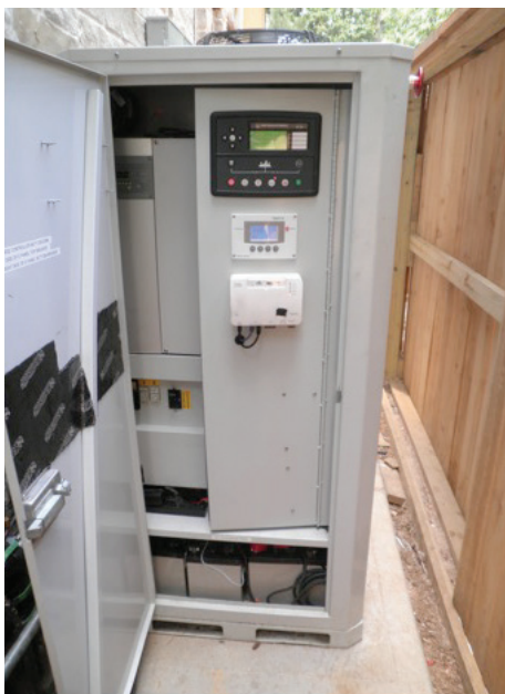
The home has the world's first tri-generation micro-generator to provide electricity, heating, and cooling in one.
