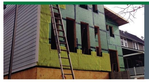
outside edge of the wall which provides adequate structural strength while leaving more room for insulation than traditional solid wood headers consisting of two 2x8s and a sheet of plywood. The wall cavities were filled with open-cell spray foam to R-20. The walls were sheathed with a coated insulated OSB and covered with a mesh rain screen to provide a ventilation gap under the fiber cement and corrugated metal cladding.
