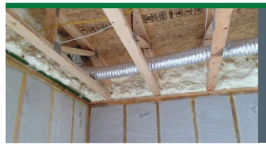
The homes' 12-inch-thick double walls are filled with 3.5-in. (R-22) of closed-cell spray foam and 8.5 in. (R-30) of blown cellulose for a total wall R-value of R-52 with no thermal bridging. The rim joists between the first and second floors are filled with spray foam to insulate and air seal this often leaky space. Open-web floor joists provide space for the ERV ducts.
