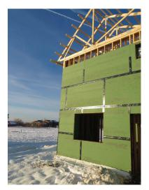
A coated OSB sheathes the exterior walls. When the seams are taped, it provides an air-sealed drainage plane and replaces house wrap, saving installation time and costs.
