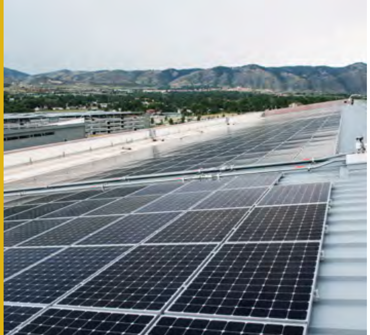
August 14, 2014 - S-5! solar panel mounting clips used on the roof of RSF-A wing.
