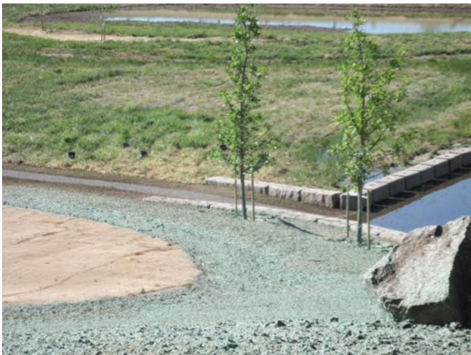
Erosion control blanket and hydromulch stormwater BMPs at the STM campus. Photo by Kurt Schlomberg, NREL/PIX 21210
