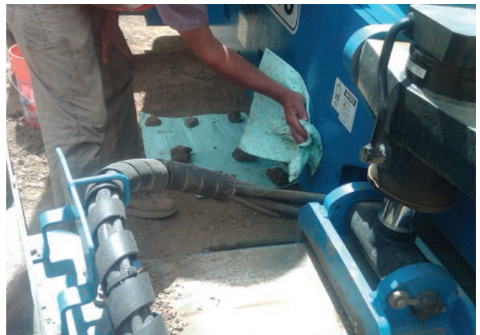
Thorough cleanup of a small hydraulic fluid leak from a boom lift. Photo by Matt Ogle, NREL/PIX 21215
