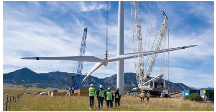
The Gamesa G9X-2.0 turbine assembled at the NWTC is the latest addition to NREL's collection of multi-megawatt wind turbines. Photo by Dennis Schroeder, NREL/PIX 20864
