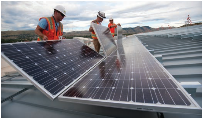
PV panel installation on the roof at the RSF. Photo by Dennis Schroeder, NREL/PIX 17843
