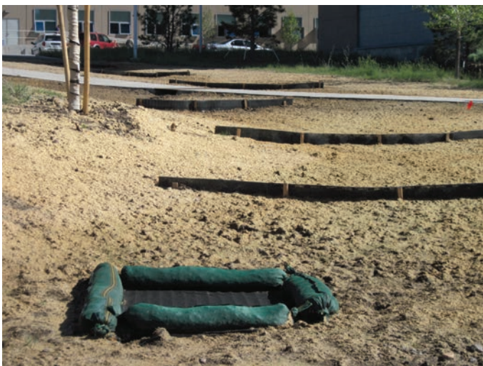
Layers of stormwater BMPs preventing erosion and controlling sediment. Photo by Kurt Schlomberg, NREL/PIX 21211
