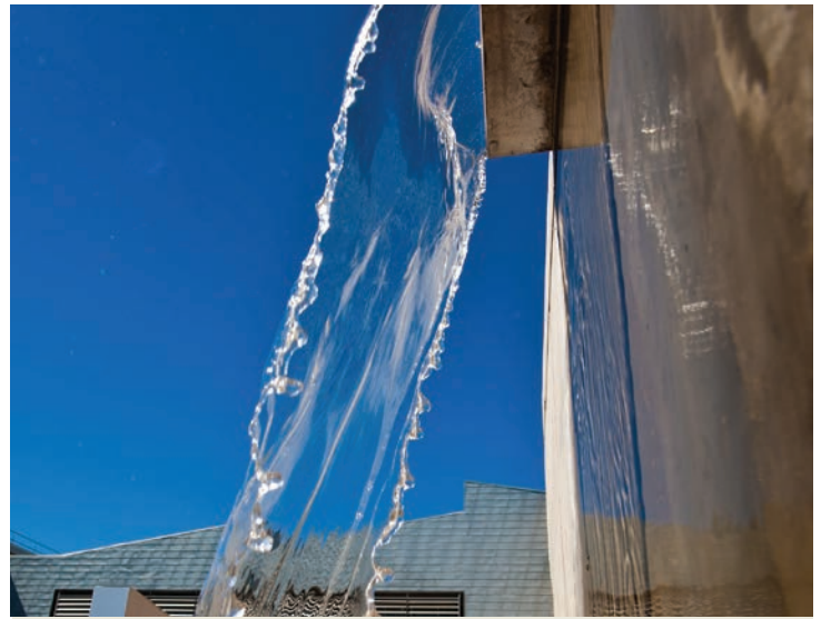
Melting snow from the roof of the RSF flows into containment structures and then into landscaping around the building. Photo by Dennis Schroeder, NREL/PIX 18640
