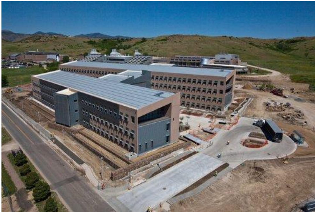
Figure 5. Research Support Facility
