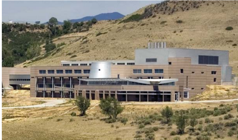
Figure 5.6. LEED platinum certified S&TF at STM
