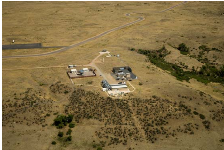
Figure 5.21. STM Site easement lands.
