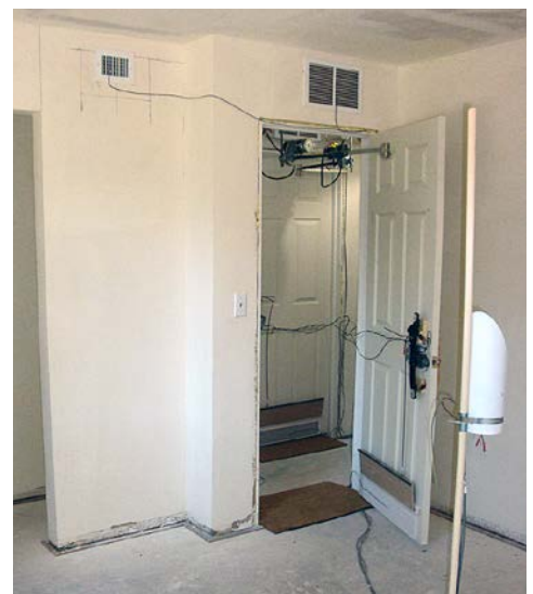
The retrofit unoccupied test house in Fresno, California, used automated doors and other equipment to facilitate testing of the high- and low-transfer grille strategy.
