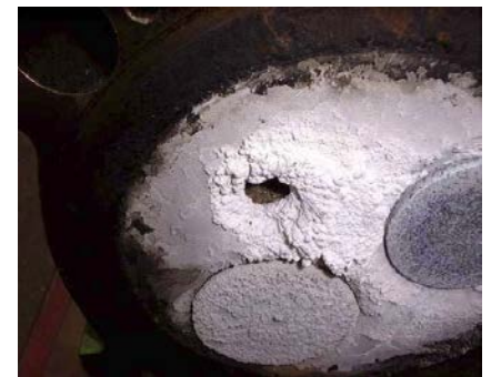
Silica deposits on engine cylinders used in CHP
