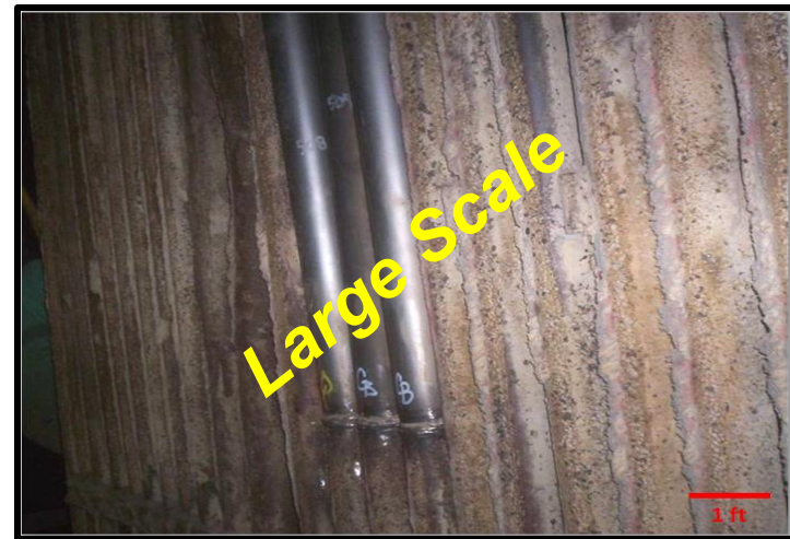
Coal Fired Power Plant, Fireside Fly Ash Corrosion Midwest Generation, Homer City, PA (still in service >3 years)
