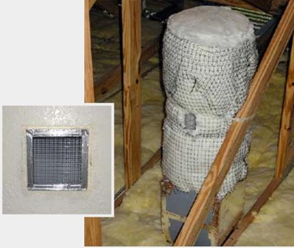
Each lab was configured with four controllable ceiling leakage sites providing ~70% of leakage area.
