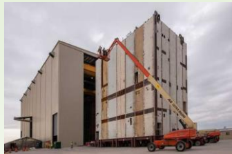
Vogtle Unit 3 CA20 module removal from module assembly building and placement on the Nuclear Island (Courtesy of Georgia Power/Southern Company)
