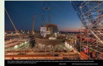
Vogtle Unit 3 CA20 module removal from module assembly building and placement on the Nuclear Island (Courtesy of Georgia Power/Southern Company)
