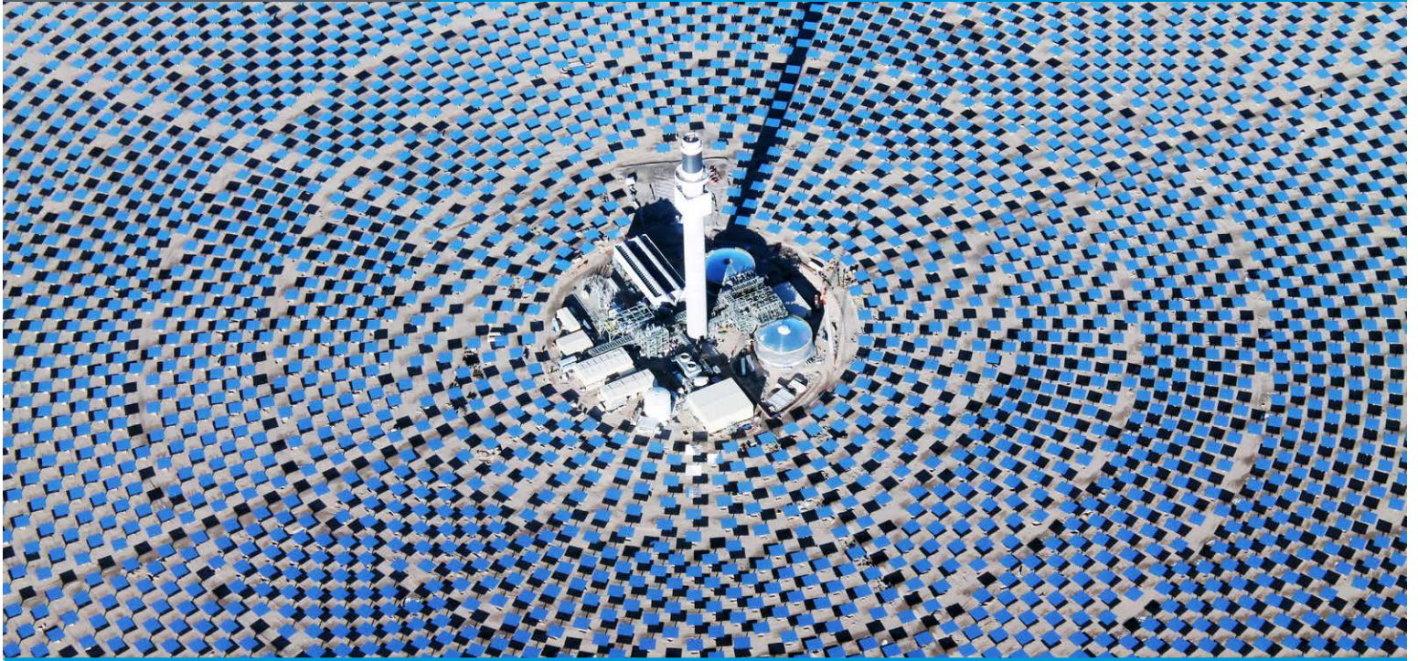
Aerial view of the Crescent Dunes 540 foot power tower in Tonopah, Nevada. Photo Credit: SolarReserve, LLC.
