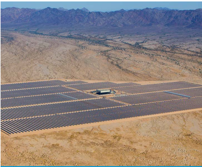
The Genesis solar energy plant is composed of two 125 megawatt parabolic trough technology units.
