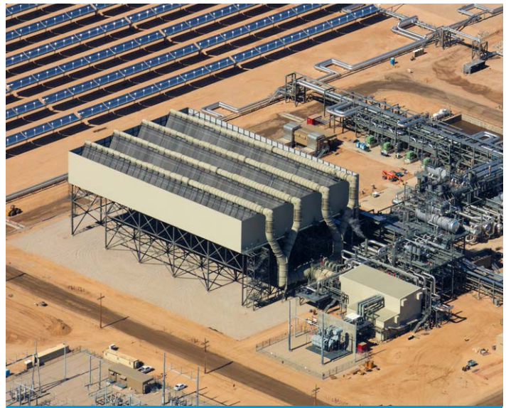
Genesis is expected to produce nearly 700 gigawatt-hours of renewable electricity each year from more than 500,000 parabolic mirrors.
