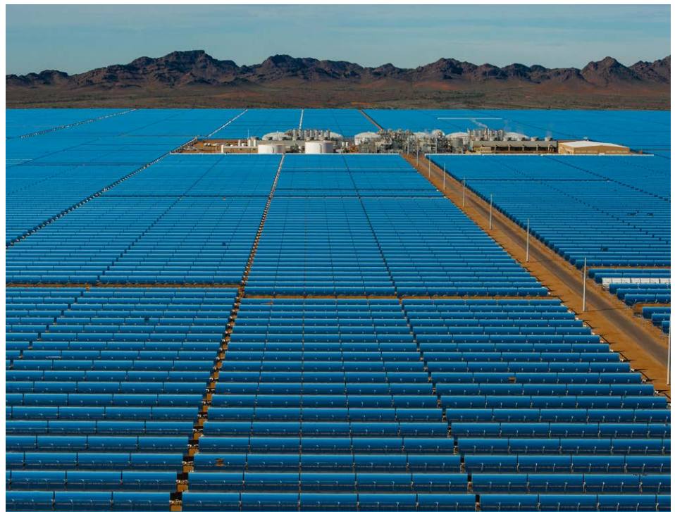
The Solana parabolic trough and thermal storage plant spans 1,920 acres near Gila Bend, Arizona.
