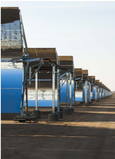
Mojave features DOE-supported parabolic trough technology to produce 250 megawatts of power. Photo Credit: Abengoa Solar, Inc.
