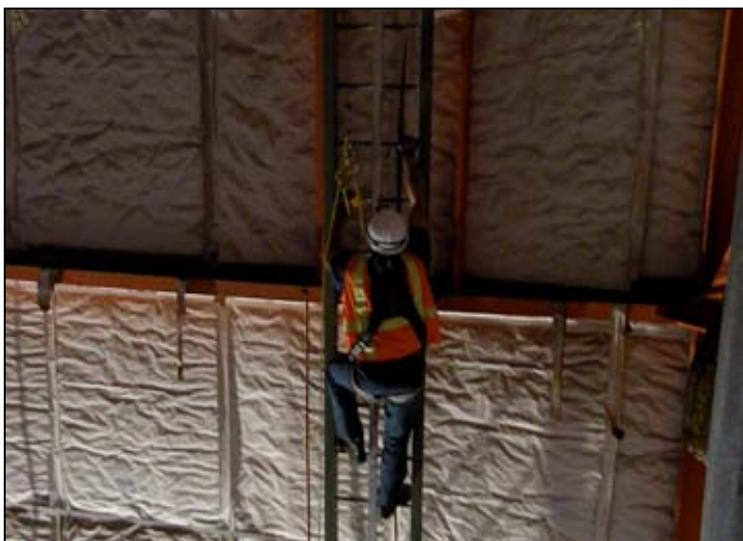
Figure 2-2. Board member ascending the ladder using retractable lanyard
