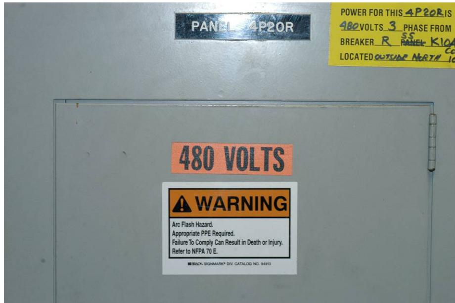
Figure 2-4. Warning label on Panel 4P20R
