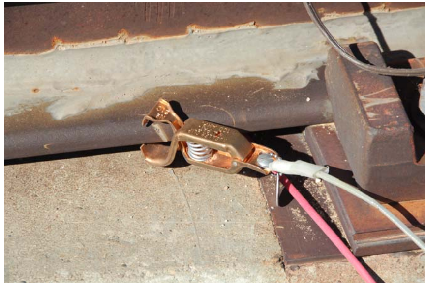
Figure 2-9. Post accident wiring to sled track (note oxidation on track rails)
