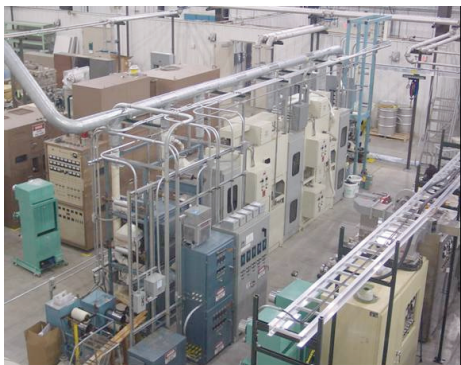
Figure 1. Conventional pilot line installation at ORNL
