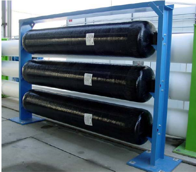
Figure 2-20 Cascade Storage Vessel Arrangement
